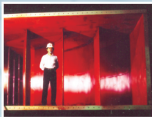
全響室迴風道出口 Exhaust Duct exit of Reverberant
