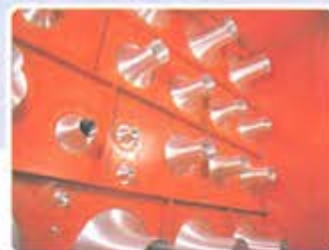
流量噴嘴 Multiple Nozzles for Flow Measurement
