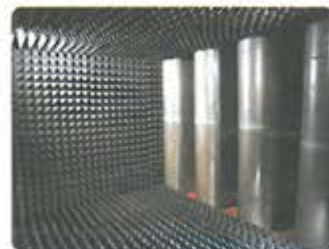
全響室迴風道裝置 Silencer in Exhaust Duct
